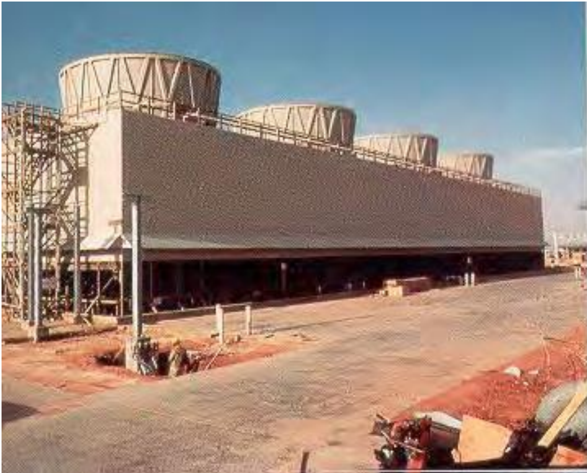
Figure 9 Counter-flow cooling tower
