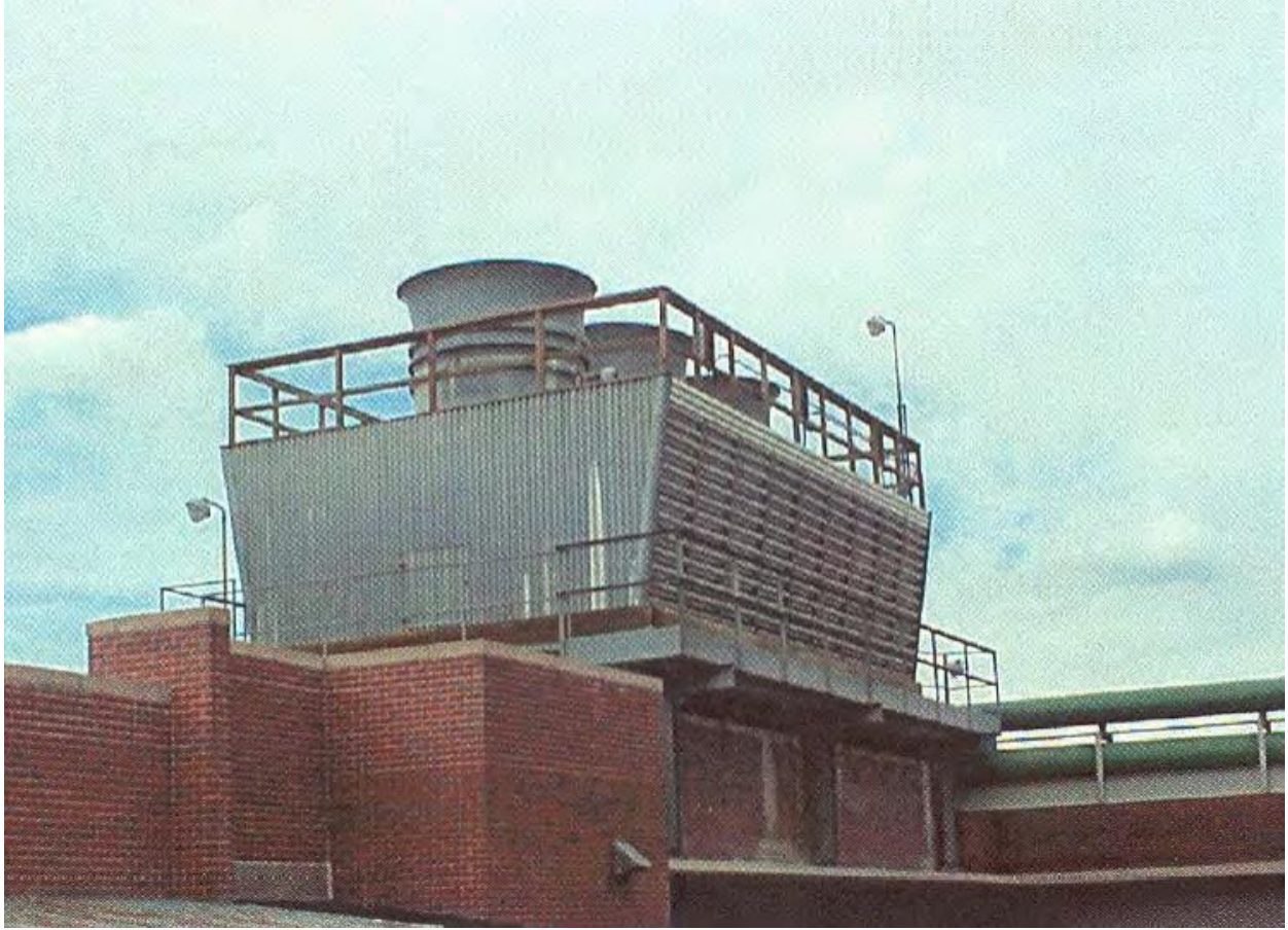
Figure 7 Cross-flow cooling tower
